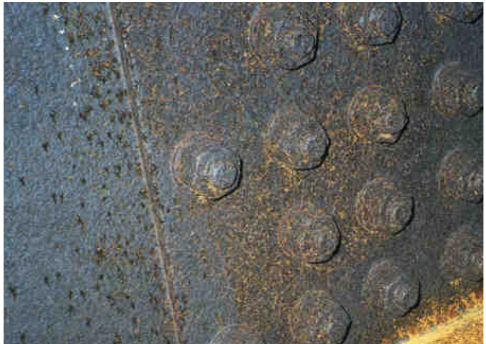
Figure 2.3.25 Chocolate Brown to Purple Brown - Boldly Exposed and Good Degree of Protection
