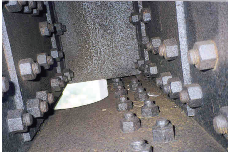
Figure 2.3.26 Black – Non-protective Oxide
