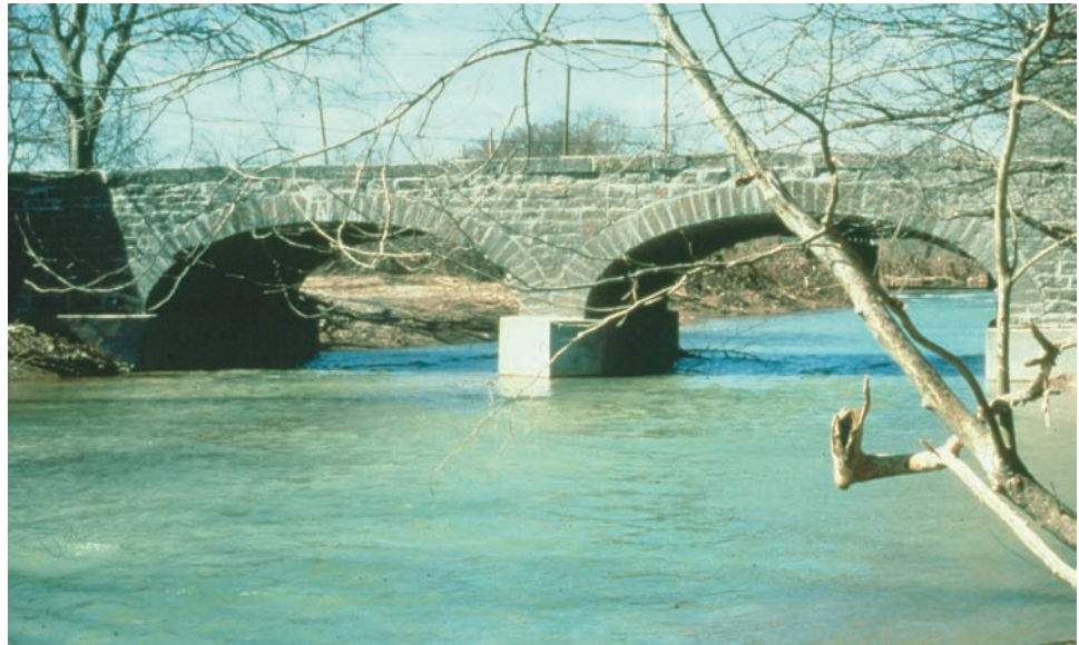
Figure 2.4.1 Stone Masonry Arch
